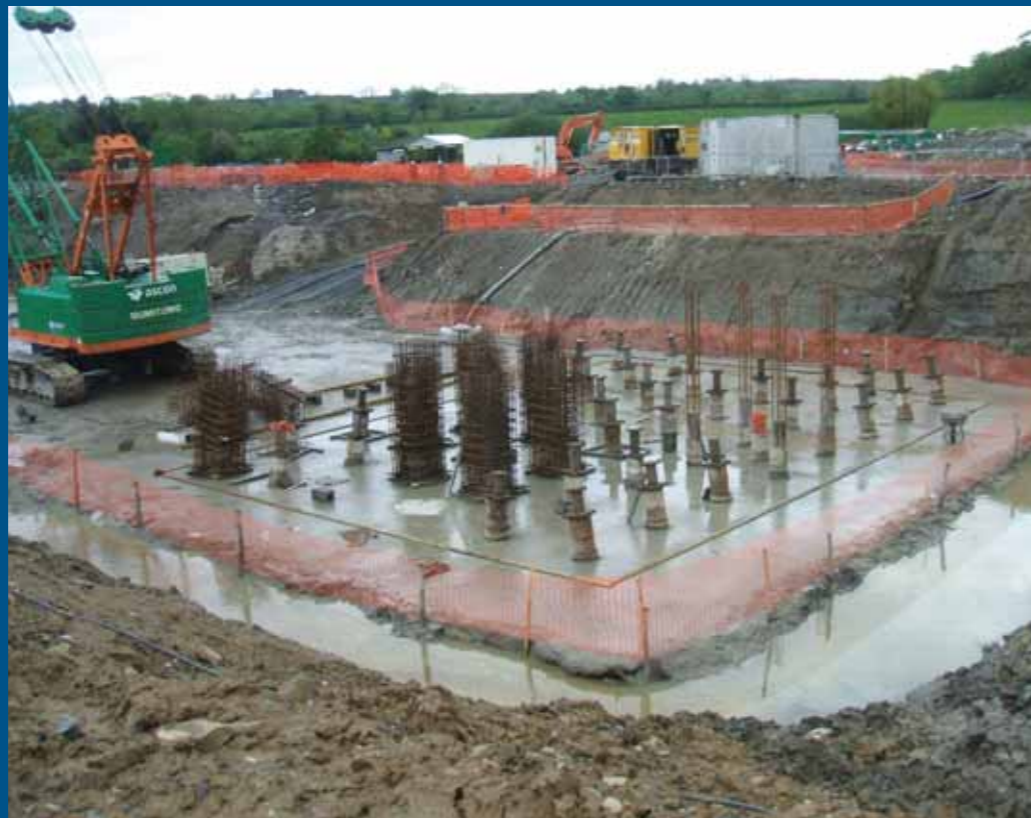
Picture shows Structure S16 – Suir Bridge
