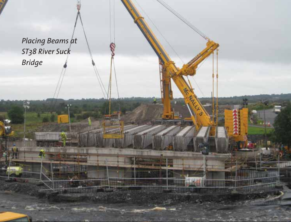
Pictured, overview of Piers and Crossheads at ST38 River Suck Bridge
