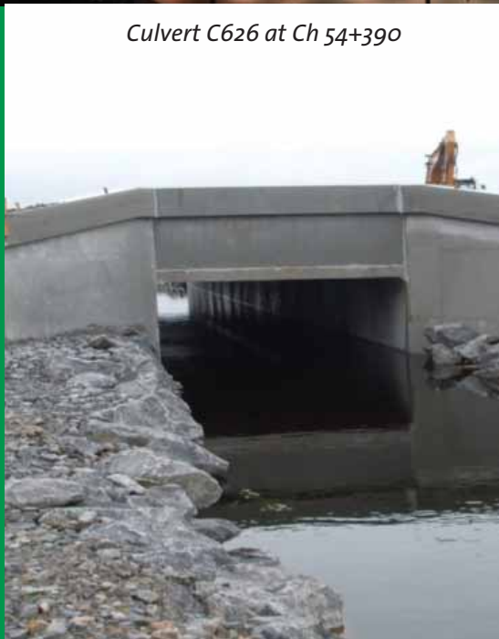
Culvert C515 Side Road at 720m (Aughrim)
