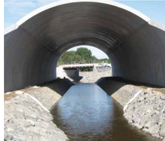
ST11 Graigabbey Overbridge with ST47 Graigabbey River Bridge 3 in the background.
