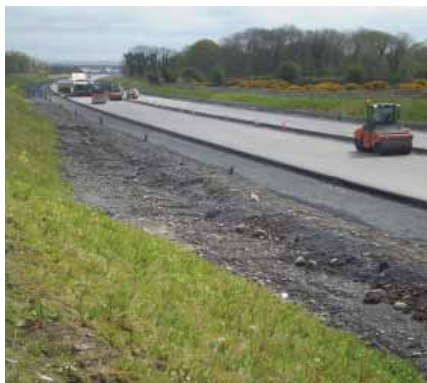
Placing of HDM basecourse (Section 1)
