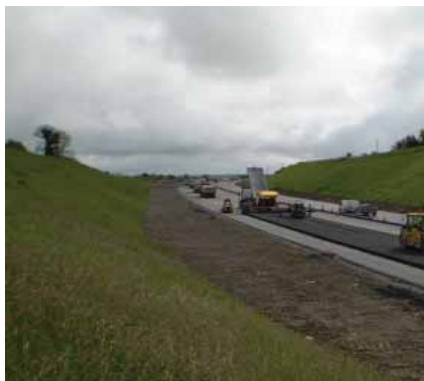
Placing of CBM Road Base (section 4)
