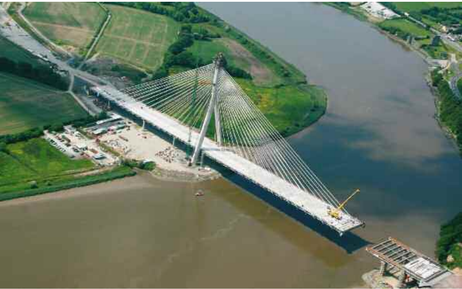
River Suir Bridge.
