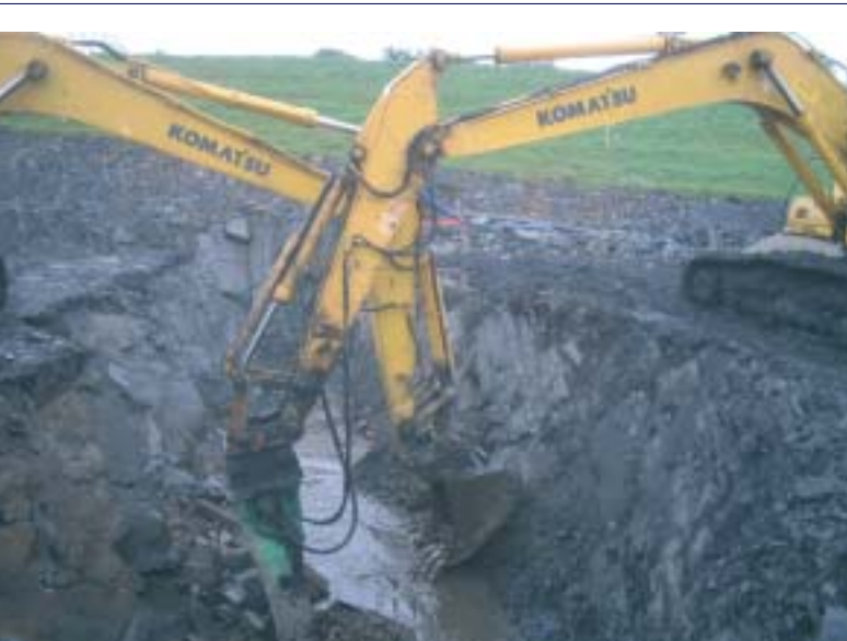
A trench is being excavated
