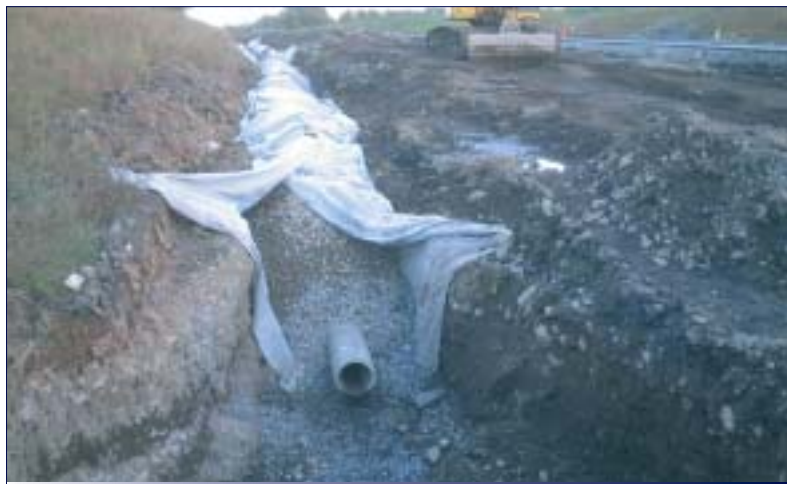
Filter drain construction
