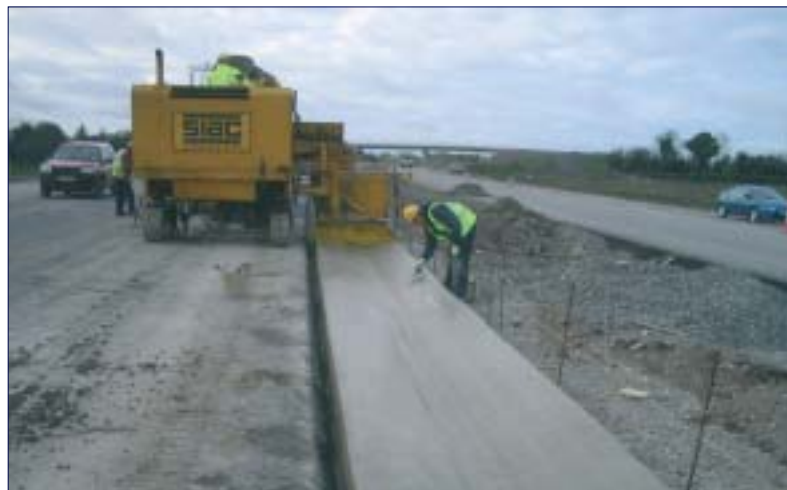
Channel is set in situ
