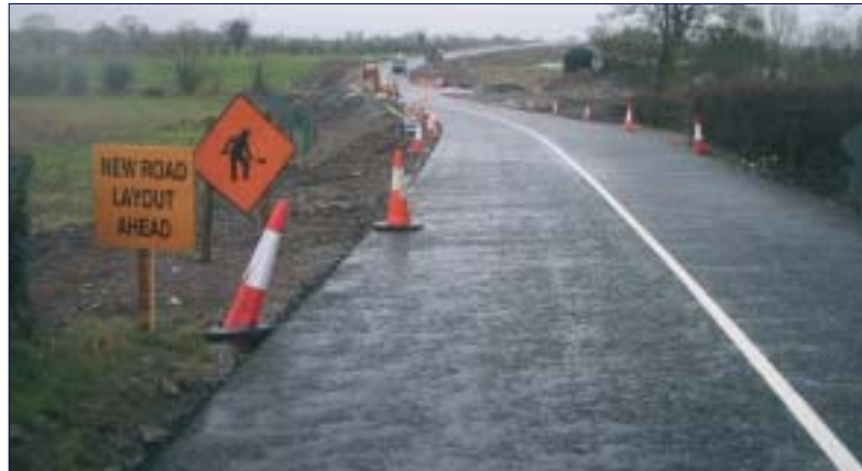
Works at side roads
