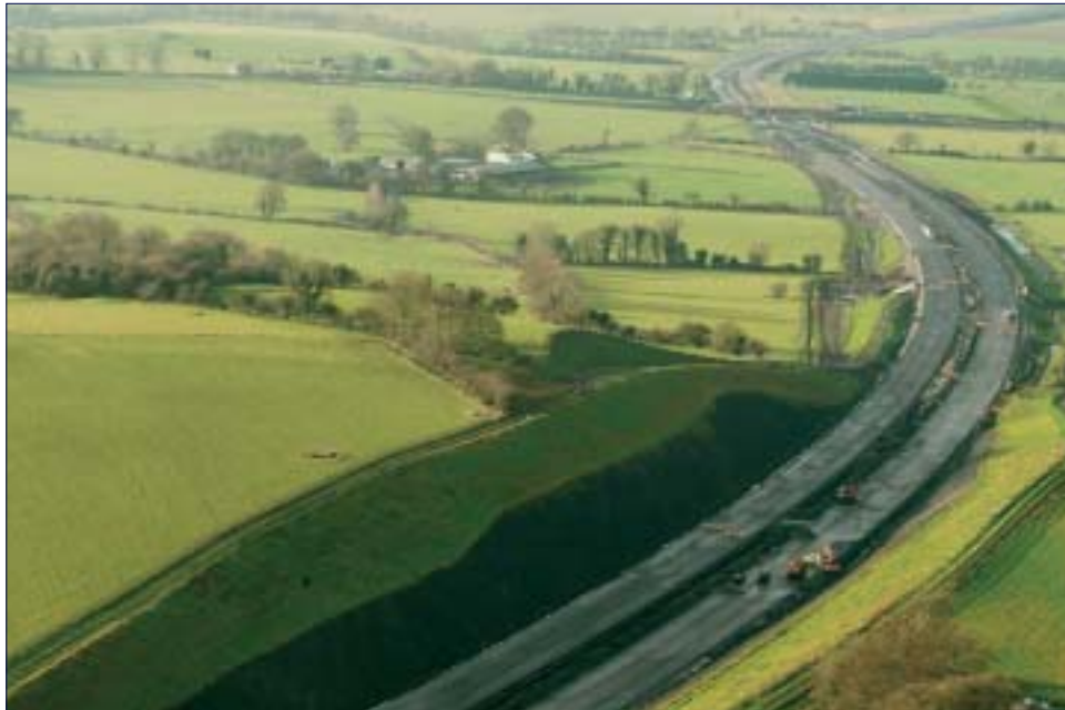
The road is sat in the natural topography
