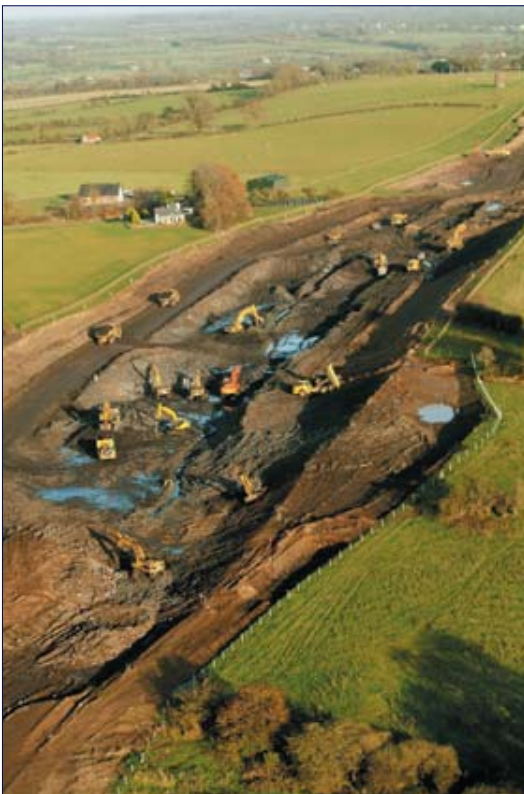
Excavation of soil and rock at Cappagh Hill
