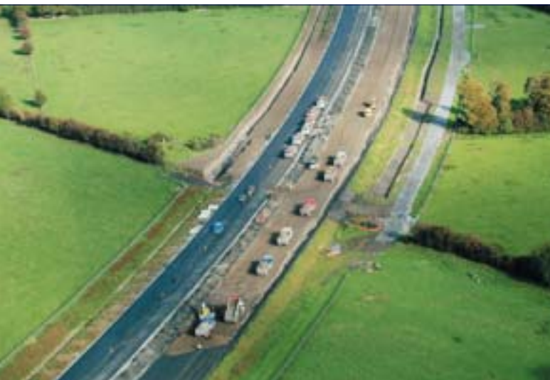
Capping operations underway
