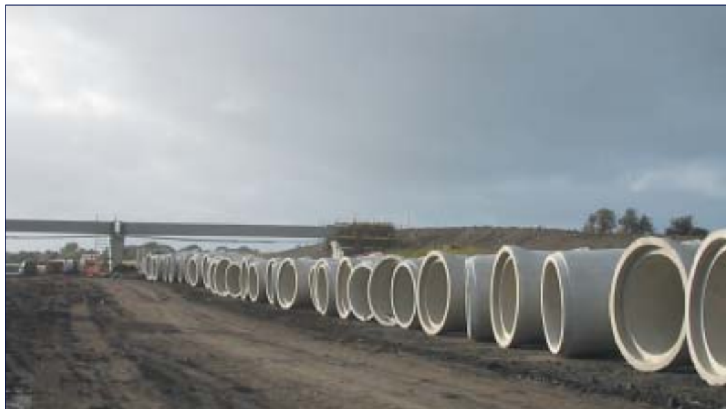
Earthworks completed to road level allow drainage to proceed
