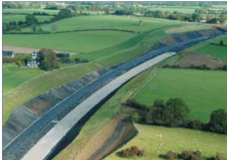
Completed earthworks at Cappagh Hill, pavement construction is underway
