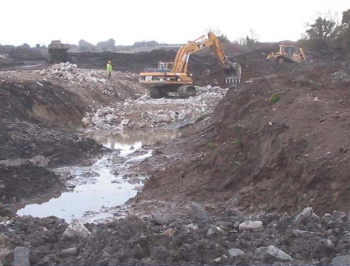
Filling a disused watercourse with rock from the site
