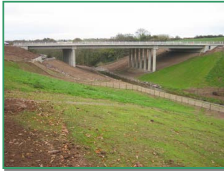
River Flesk Bridge S05, Looking East
