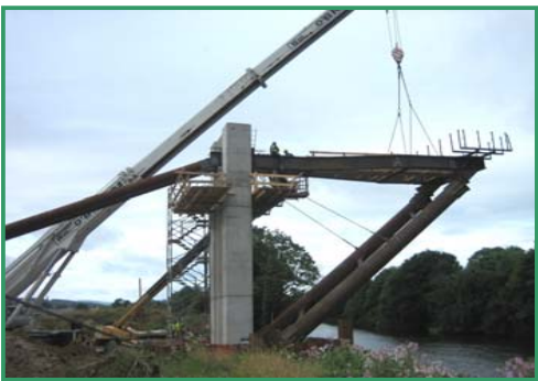
Temporary works for launching deck
