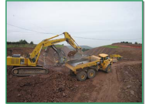
Removal of Earthworks "Plug" at Rathcormac South Interchange, Looking North
