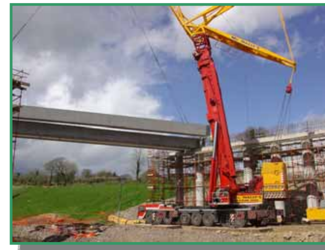
Placing precast beams to the River Flesk bridge
