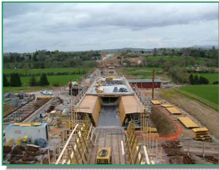
Launch of the second deck segment underway, looking north.
