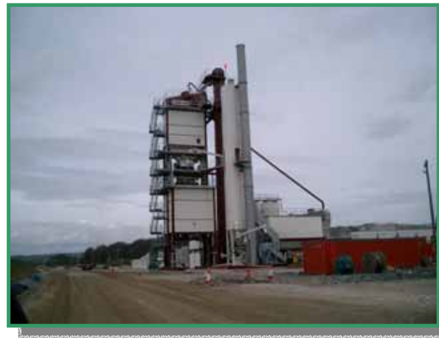
View of temporary Asphalt Plant used to manufacture pavement materials
